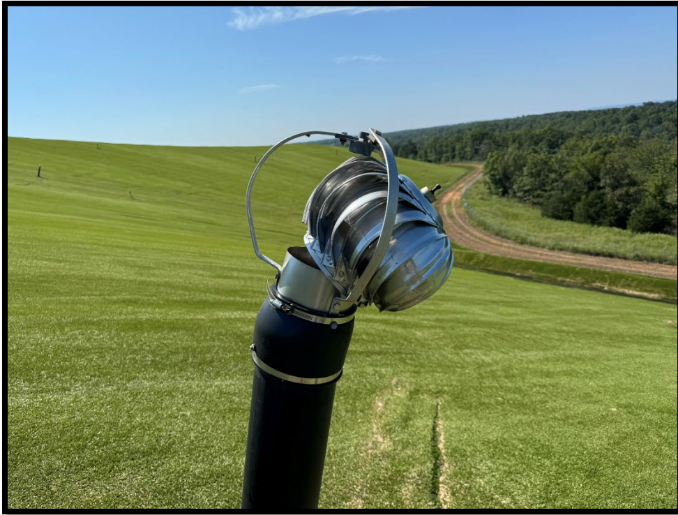
Photograph 3: View of damaged turbine vent on north side of Area 1-2.
