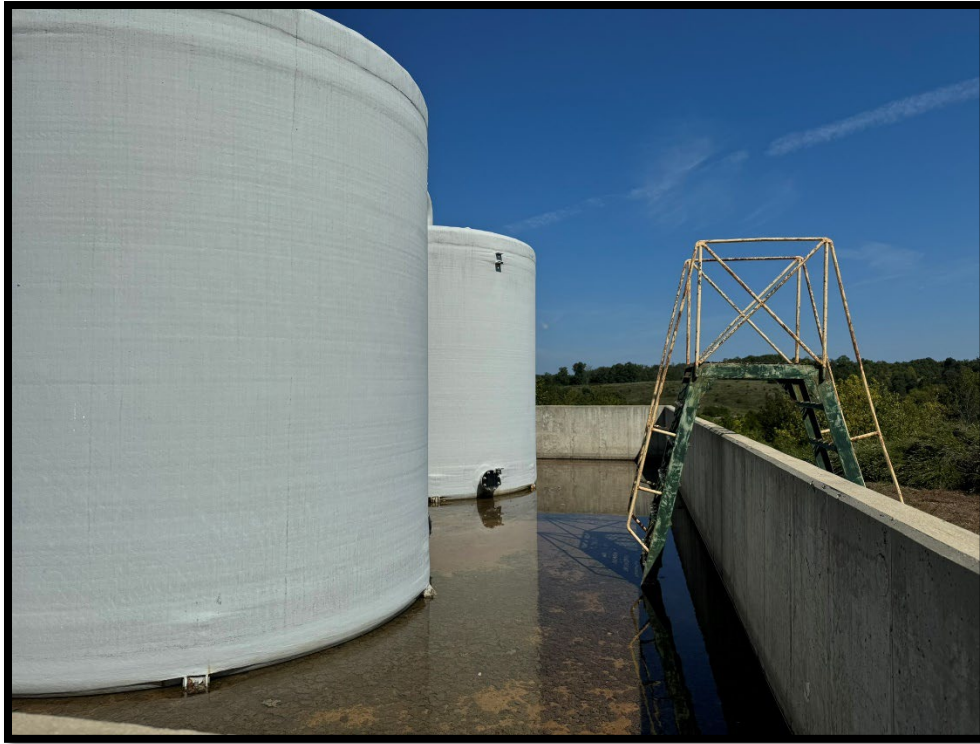
Photograph 1: View of minimal stormwater in leachate tank battery.
