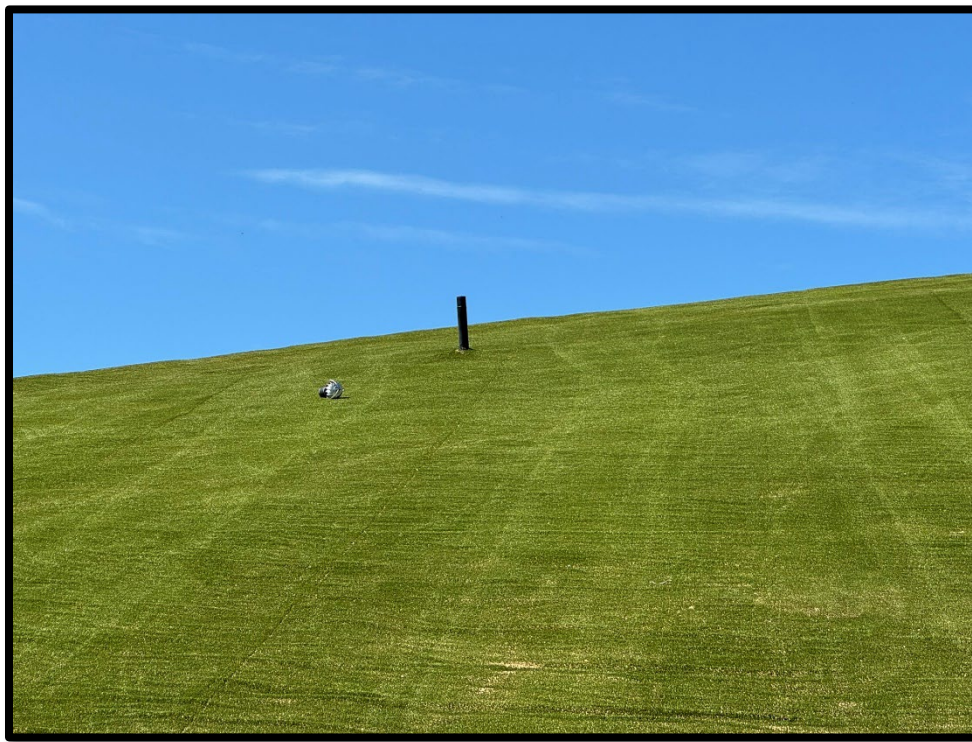
Photograph 2: View of detached turbine vent near LCS-8.
